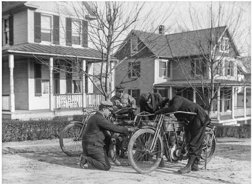
In 1916, Maryland's Supreme Court overturned a law that cited fire hazards as justification for outlawing brick apartments near wood-framed single-family homes.
